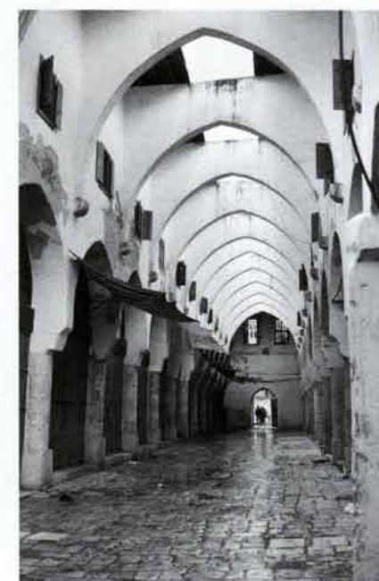
One of few khans to be restored in Lebanon, Tripoli's Khan al-Khayyat (Tailors' Khan) is also an unusual example of a khan that may have been built not around a courtyard, but by roofing over a much older street.
